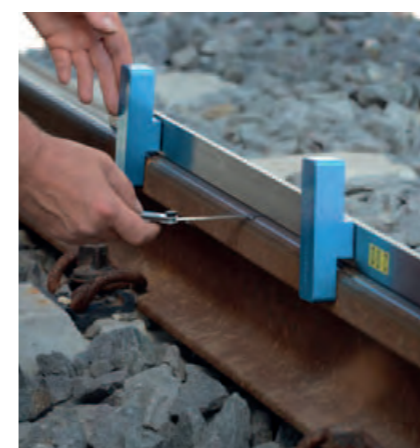
Inspecting rail straightness
