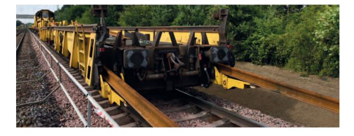
Fully automatic: Long rails are gripped securely and placed directly on the sleeper heads or in the middle of the track
